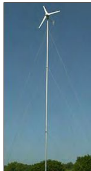
Figura 3: Torre con riendas (Wind Turbine Towers)
