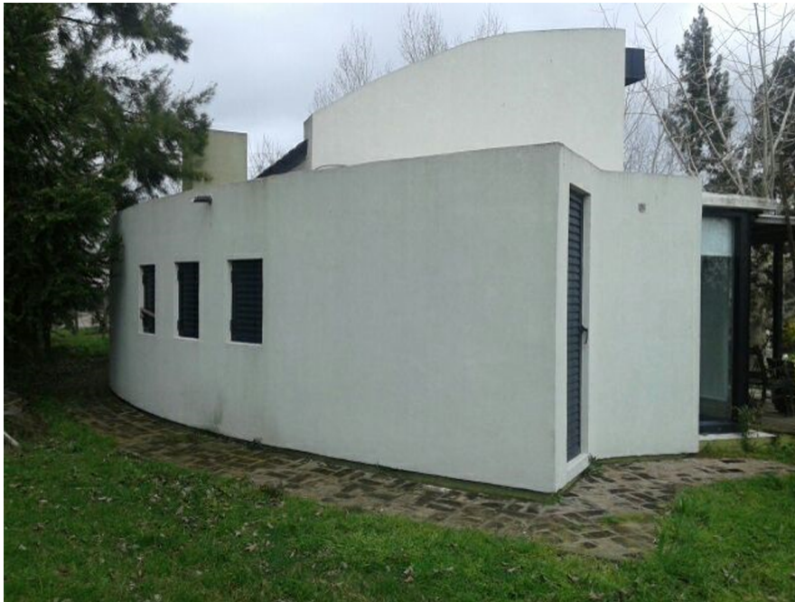
Fig. 1 Refurbished wall Southern view
