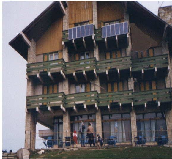
Fig. 3b PV-Powered Emergency Signal Repeater Station
