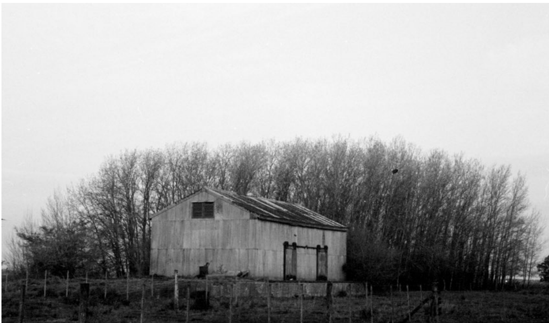
Grain silo in Vergara, Buenos Aires Province. Ferrocarril del Sud, 1921 (photo by author)
