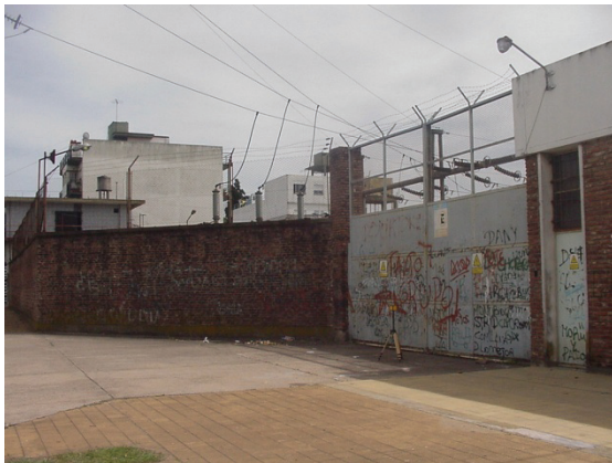
Figure 8: Measurement in a Substation (SE23)
