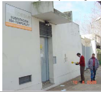
SE22: linkage only underground
