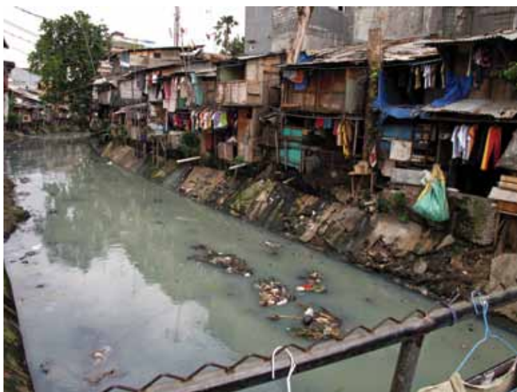
PHOTO 2.1 Difficulties implementing known and even low-cost solutions. Cleaning clogged drainage systems would mitigate the risk of flooding. However, such well-identified and cost-effective solutions often fail to be implemented. The Mumbai case illustrates a common problem (as seen in this picture from Jakarta).
