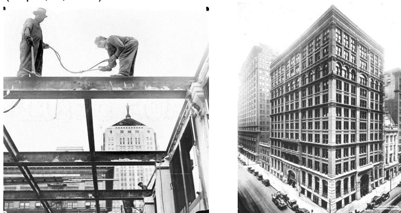
Figuras III – 1 y 2: Edificio de la Home Insurance, Chicago (1885) – Fuente: United States Library of Congress's National Digital Library Program – Disponible en: http://memory.loc.gov
