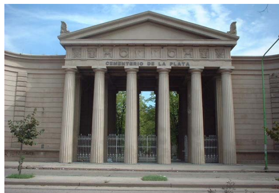
Fig. 1.3. Entrada principal del CMLP.
