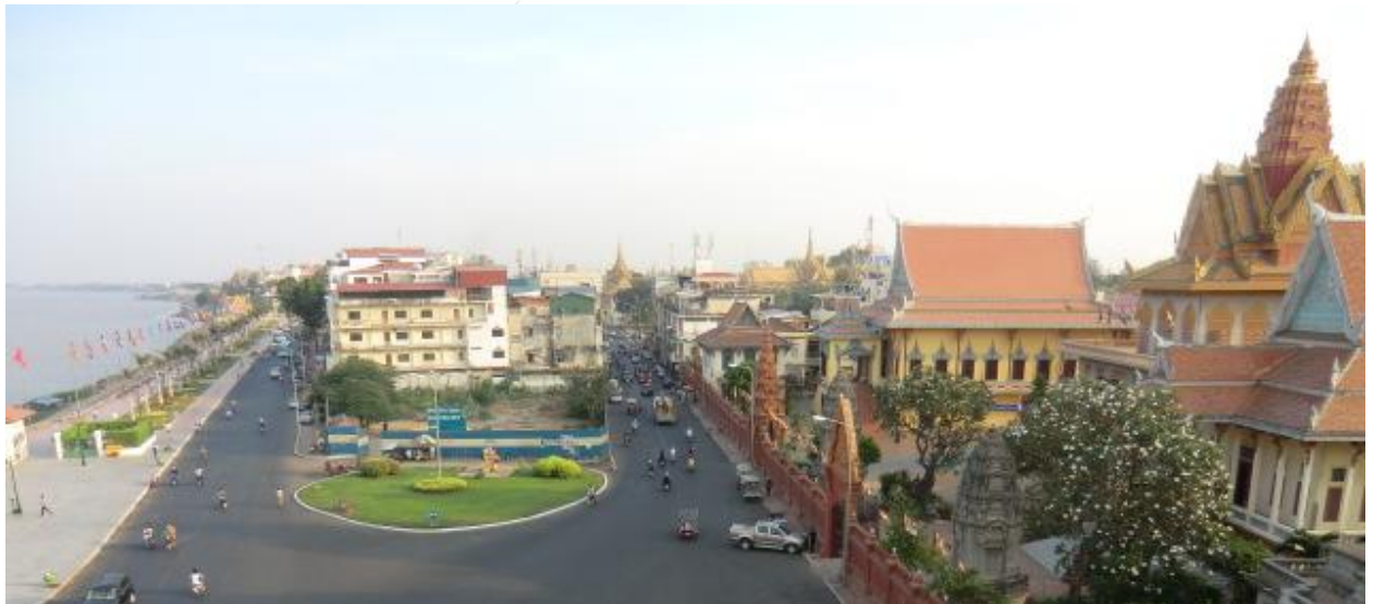
Photo 4.2 Phnom Penh – City Centre near the Tonle River
