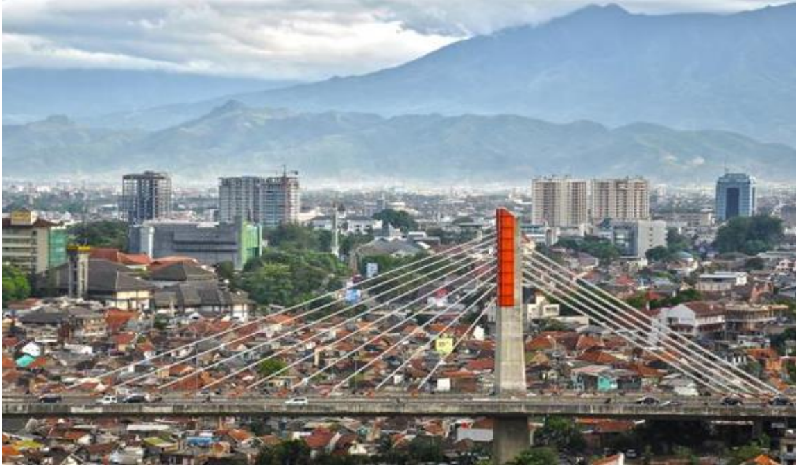
Photo 3.1 Pasupati Bridge, Bandung City
