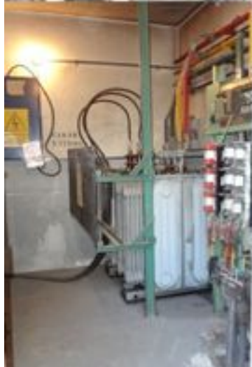
Compaction OHL-MV/LV Substations
