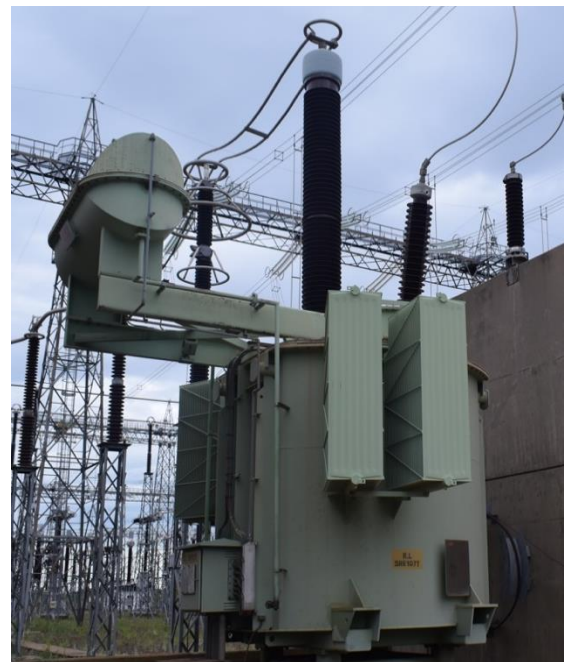
Fig. 6. Caso 4: 500 kV – 26.67 MVar (reactor monofásico)
